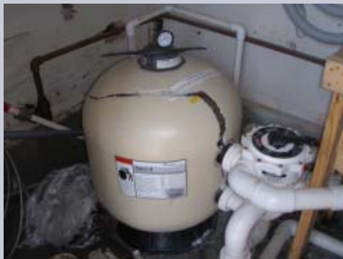
Pool was not winterized properly resulting in a cracked filter tank and plumbing lines.
